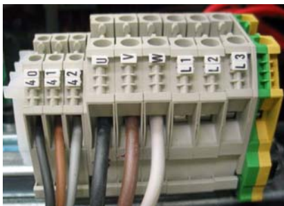
Fig. 21: Power supply terminal board
